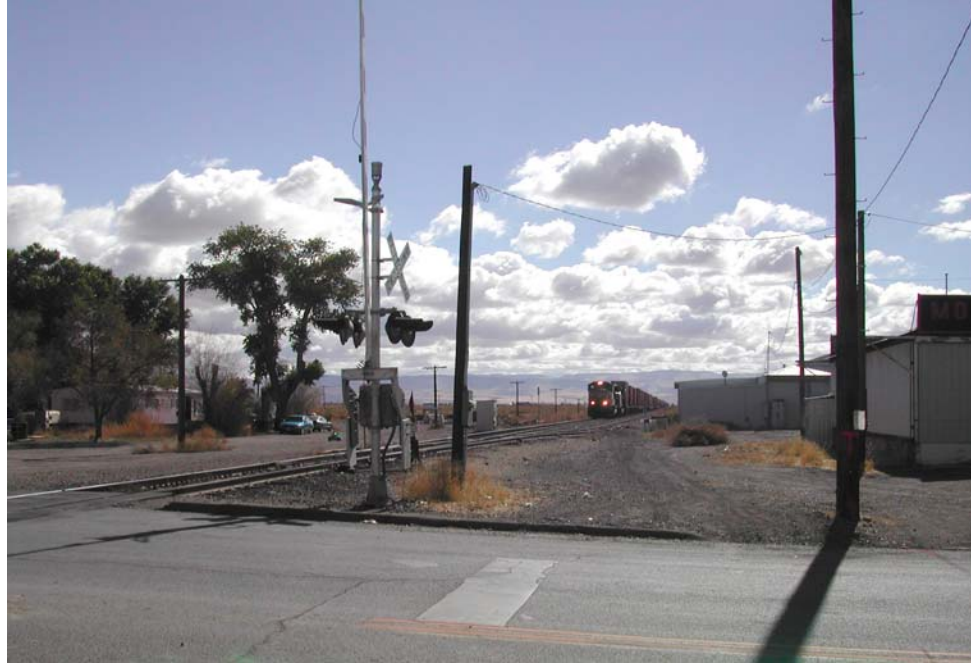
Figure 11: Active Siding east of Reese Crossing
