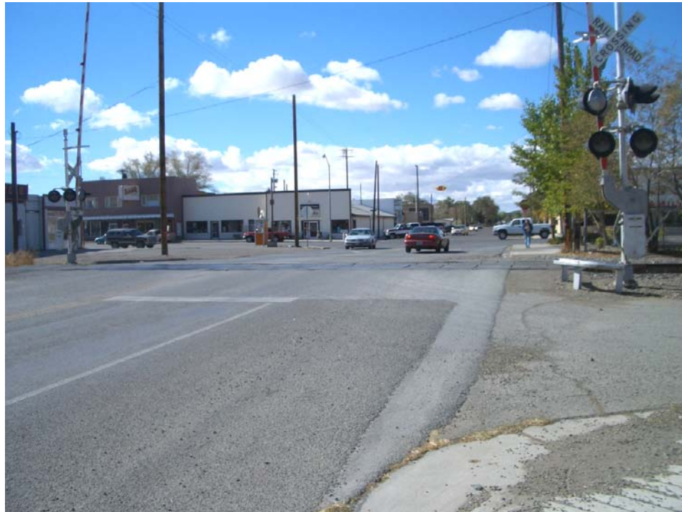
Figure 10: Reese Street Crossing Track No. 1 - View looking south towards Front Street, which is parallel to the track
