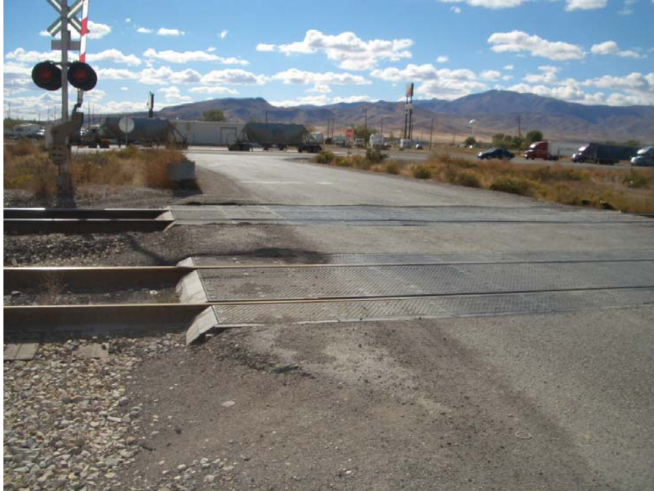
Figure 9: Rubber Crossing Panels at North Second Street- view looking south
