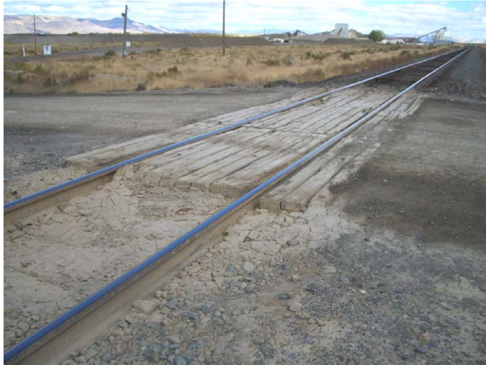
Figure 13: Baker-Hughes-INTEQ Crossing – looking towards the facility –View shows timber panels and deteriorated track substructure
