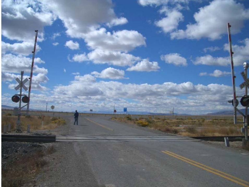
Figure 12: Muleshoe Ranch Road Crossing Track No. 1 – View looking south towards I-80
