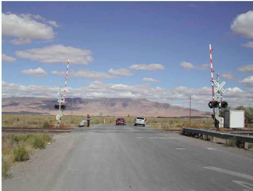
Figure 8: North Second Street crossing Track No 1 –View looking north
