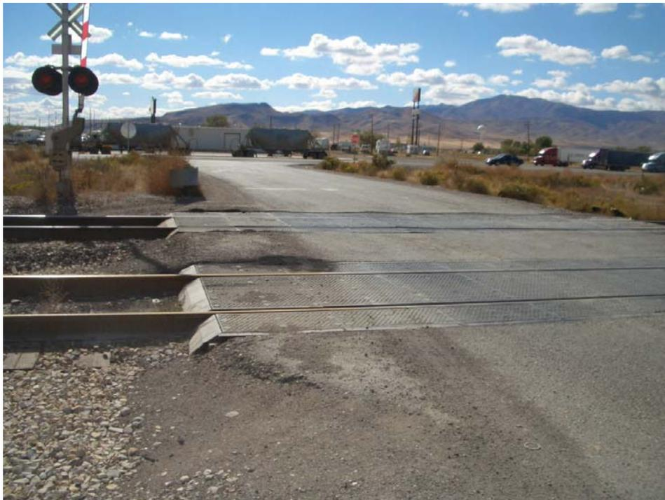
**Figure 8 Rubber Crossing Panels at North Second Street- View Looking South**
