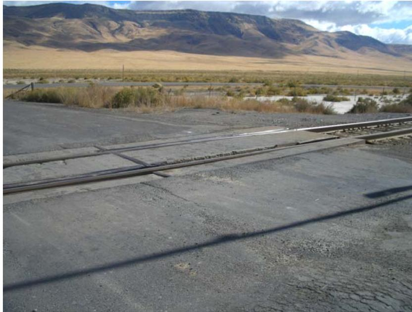
**Figure 4 Concrete Crossing Panels through the Paved State Highway 35
