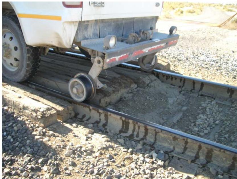
**Figure 2 Timber Panels on Track No. 2 Eastward at Mote Road Crossing**
